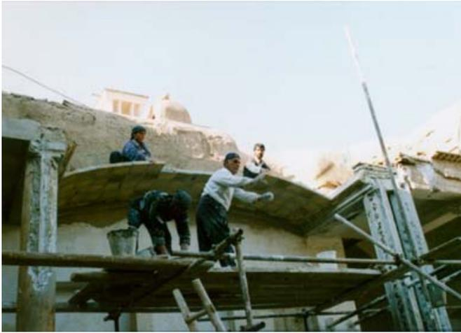
Figure 5: Implementation of Lapoosh arch by a mason and his two apprentices [14].
