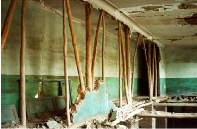
Figure 13: Using diagonal and vertical bracings inside walls. [14]
