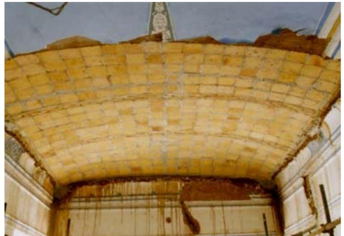
Figure 4: Lapoosh or Ghomipoosh arch used in the roof of an Iranian house[14].
